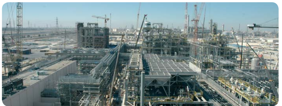
Hostalen ACP and Lupotech T process plants under construction at Al-Jubail
