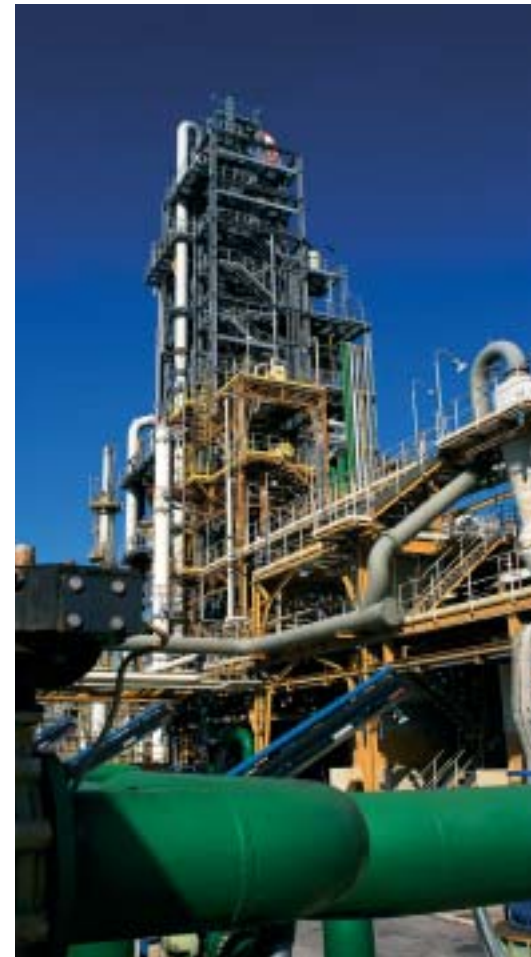
Spherizone process plant in Brindisi, Italy
