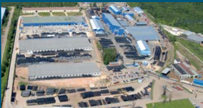
Klimovsk pipe plant
