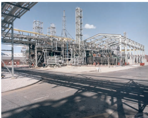
Figure 2. LyondellBasell's LDPE unit in Carrington, UK, based on Lupotech T technology
