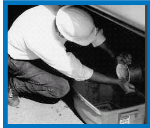
Figure 11. Hopper car delivery: inspecting the unloading tube and placing a filter and catch pan.
