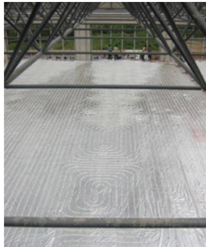
Fig. 8 – Underfloor heating made from Hostalen 4731 B – courtesy of Kingbull
