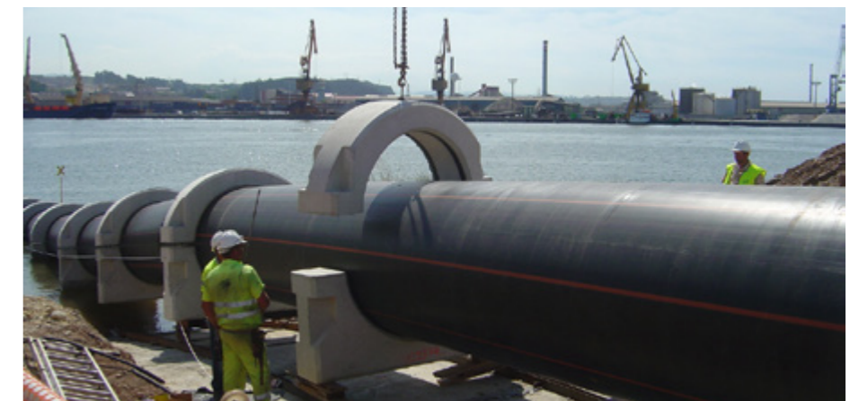
Fig. 5 - Seaoutfall line - courtesy of PLOMYPLAS
