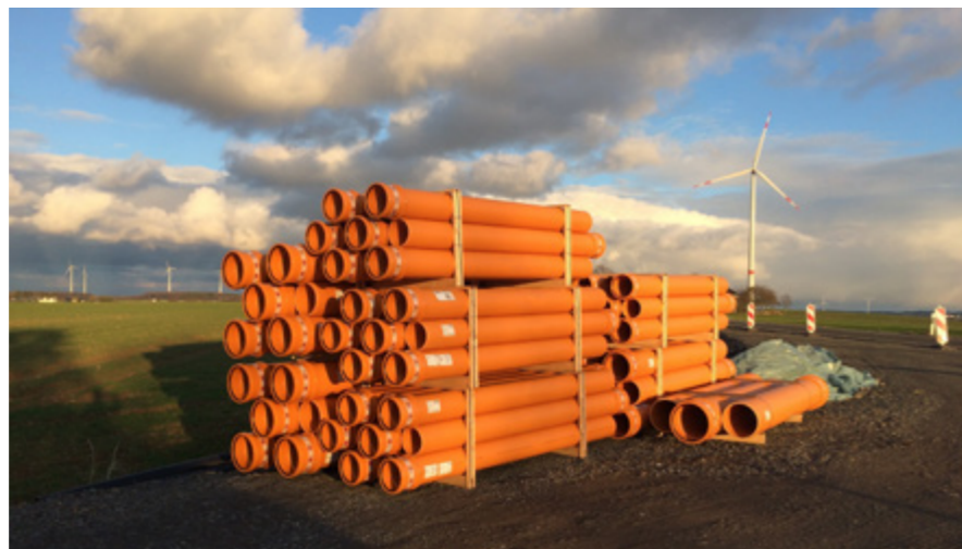
Fig. 15 - 375mm and 400mm orange sewage pipes waiting to be installed
