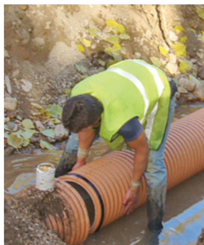
Fig. 16 - Push connection, inline socketing courtesy of PLOMYPLAS
