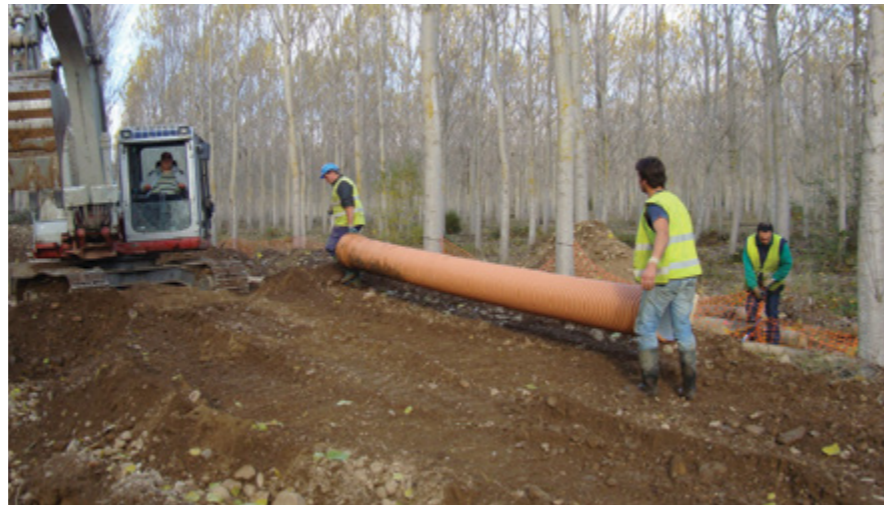
Fig. 14 - Corrugated pipes made from Hostalen PP H2464 - courtesy of PLOMYPLAS
