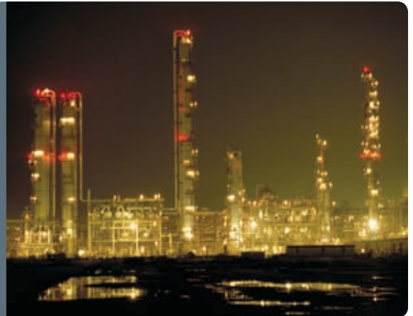
Vacido plant – LyondellBasell, La Porte, Texas, USA
