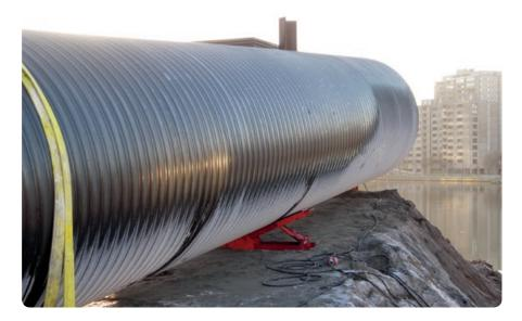
Cover: Large Weholite® pipes (DN/ID 2000 mm) connect the heat-pump plant to the sea. These pipes are produced from the LyondellBasell multimodal PE 80 material *Hostalen* GM 5010 T3 black resins and can be permanently connected from inside by extrusion welding. The welder is therefore protected from outside weather conditions – important for rapid completion of the project in the harsh Finnish winter.
