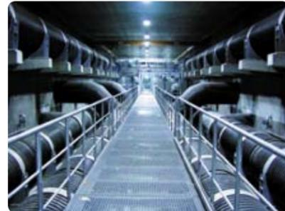
Fig. 1: View of pipe installation walkway with DN 1000, DN 1200 and DN 1400 pipelines
