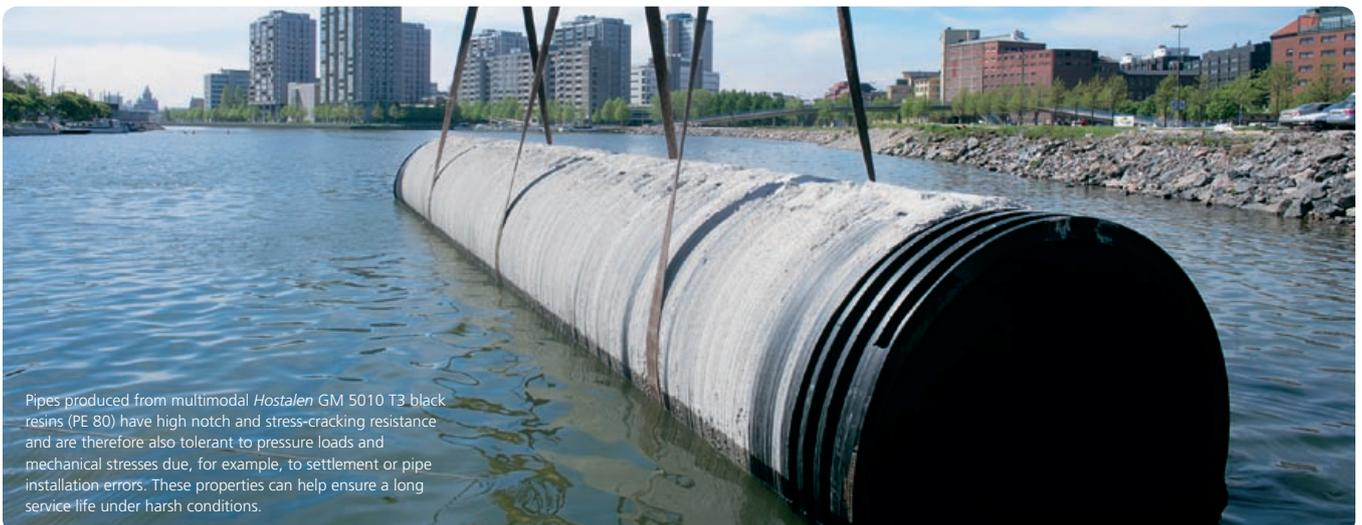
Pipes produced from multimodal *Hostalen* GM 5010 T3 black resins (PE 80) have high notch and stress-cracking resistance and are therefore also tolerant to pressure loads and mechanical stresses due, for example, to settlement or pipe installation errors. These properties can help ensure a long service life under harsh conditions.
