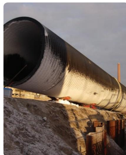
**Cover:** Large Weholite® pipes (DN/ID 2000 mm) connect the heat-pump plant to the sea. These pipes are produced from the LyondellBasell multimodal PE 80 material *Hostalen* GM 5010 T3 black resins and can be permanently connected from inside by extrusion welding. The welder is therefore protected from outside weather conditions – important for rapid completion of the project in the harsh Finnish winter.
