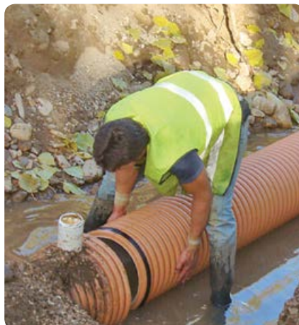
Fig. 16 – Push connection, inline socketing courtesy of PLOMYPLAS
