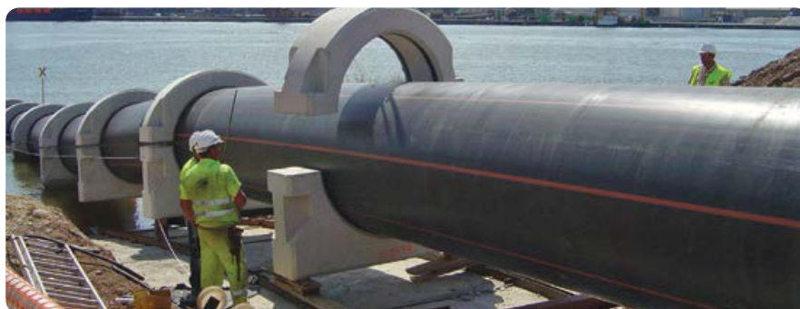
Fig. 5 – Seaoutfall line – courtesy of PLOMYPLAS
