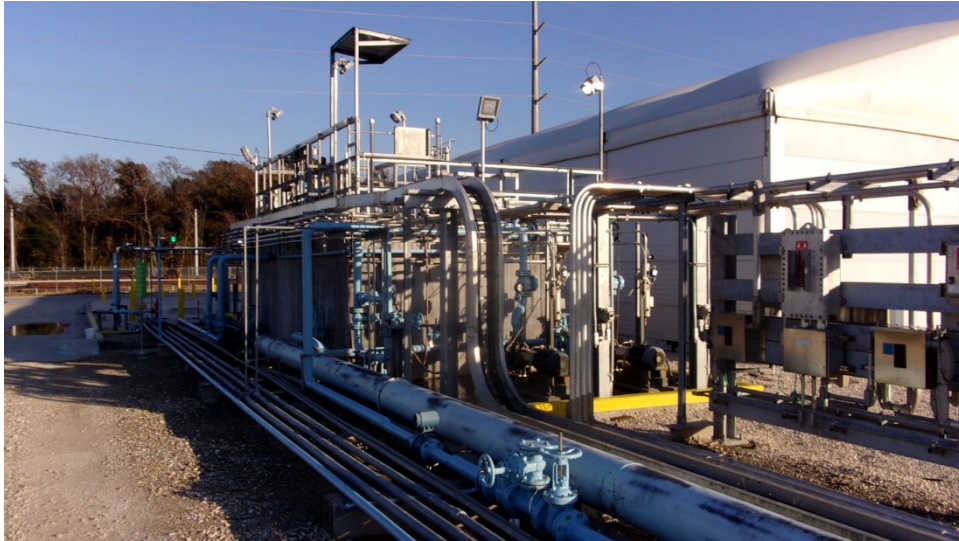
20. Outfall 201 septic chlorinator
