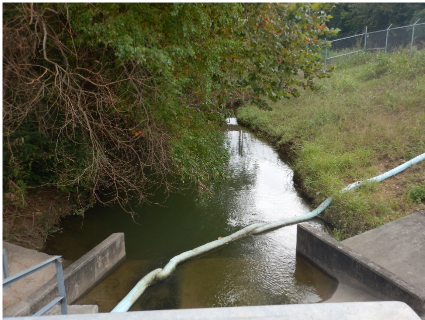
4. Outfall 002 looking downstream from discharge structure
