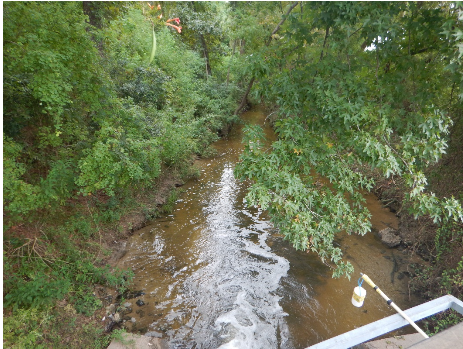
2. Outfall 001 looking downstream from sample point
