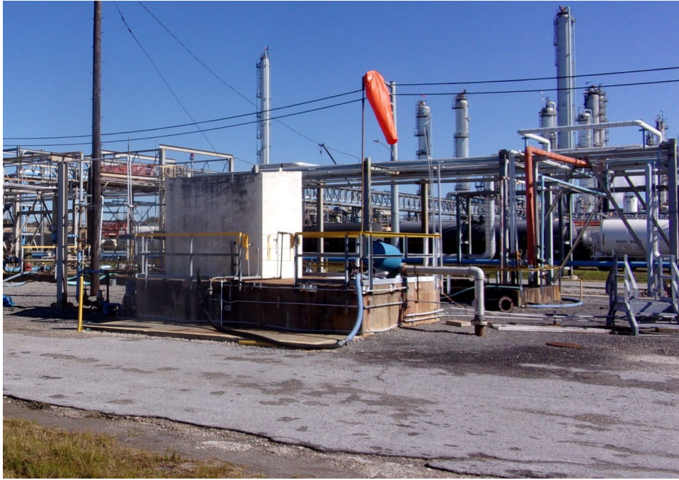
19. Outfall 101 septic chlorinator
