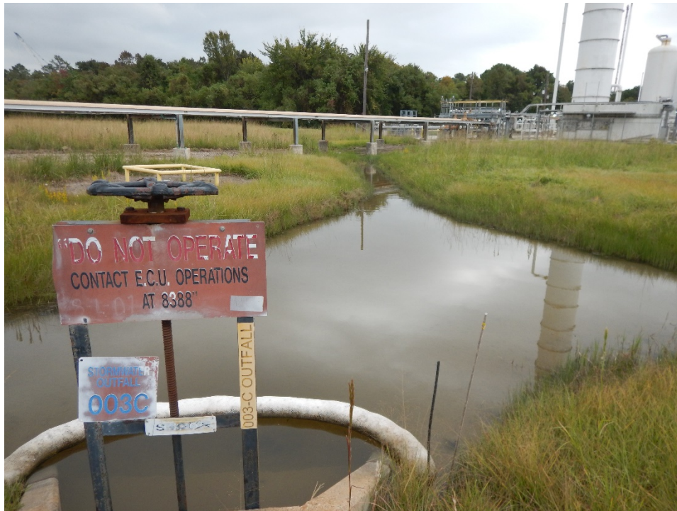
12. Outfall 003C looking downstream, outfall discharge valve lower left.
