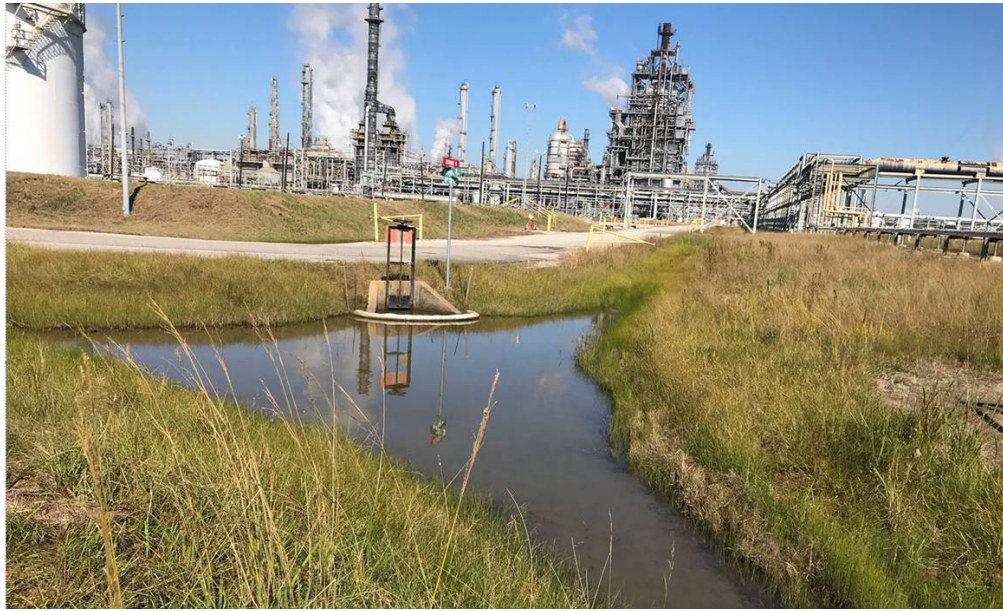
11. Outfall 003C discharge structure (center)
