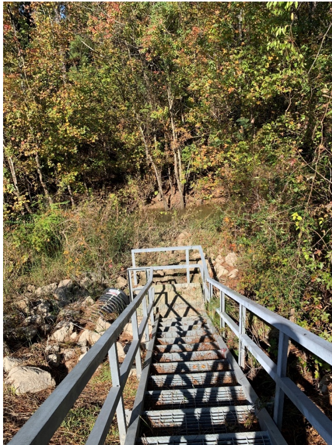
18. Outfall 006 stairs to discharge pipe, HCFCD ditch past stairs, photo center
