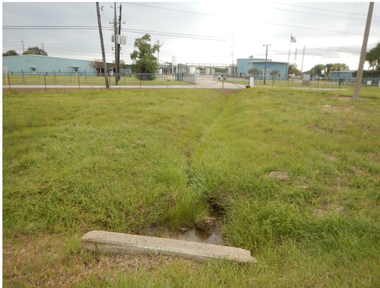
8. Outfall 003A looking downstream, outfall structure bottom center
