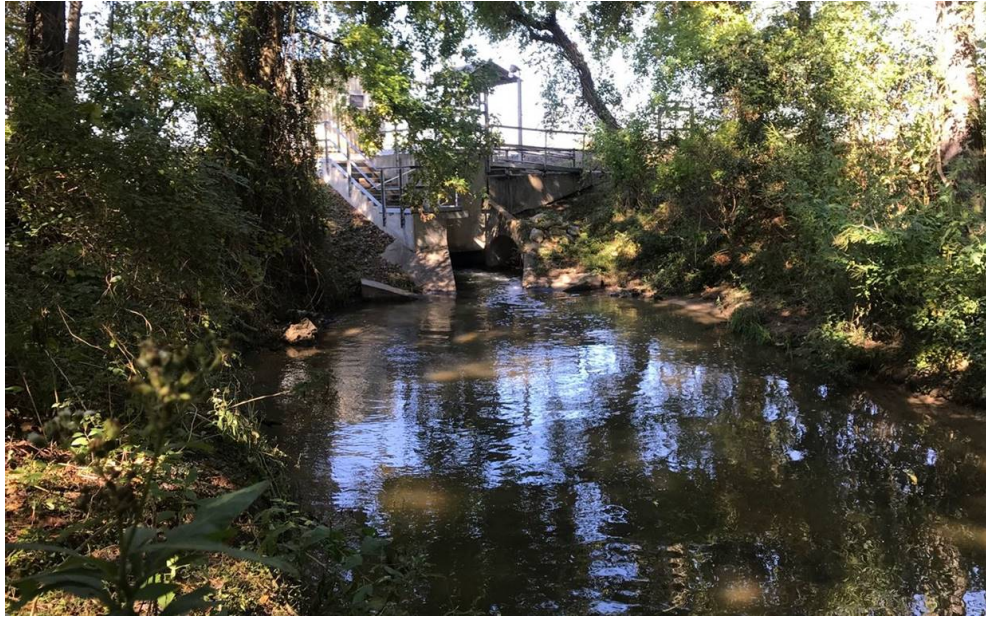
1. Outfall 001 discharge structure (upper center), discharge and channel in foreground
