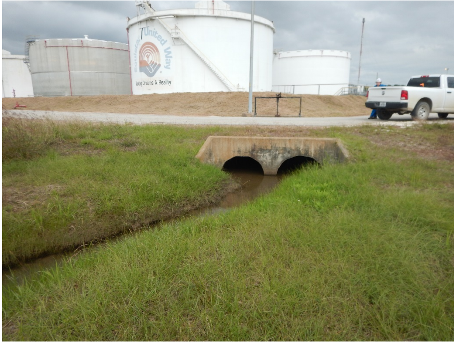
5. Outfall 003 discharge point
