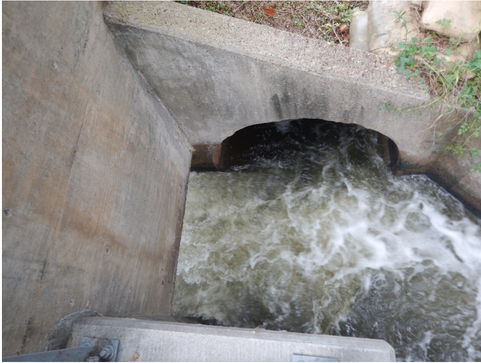
13. Outfall 004 discharge point
