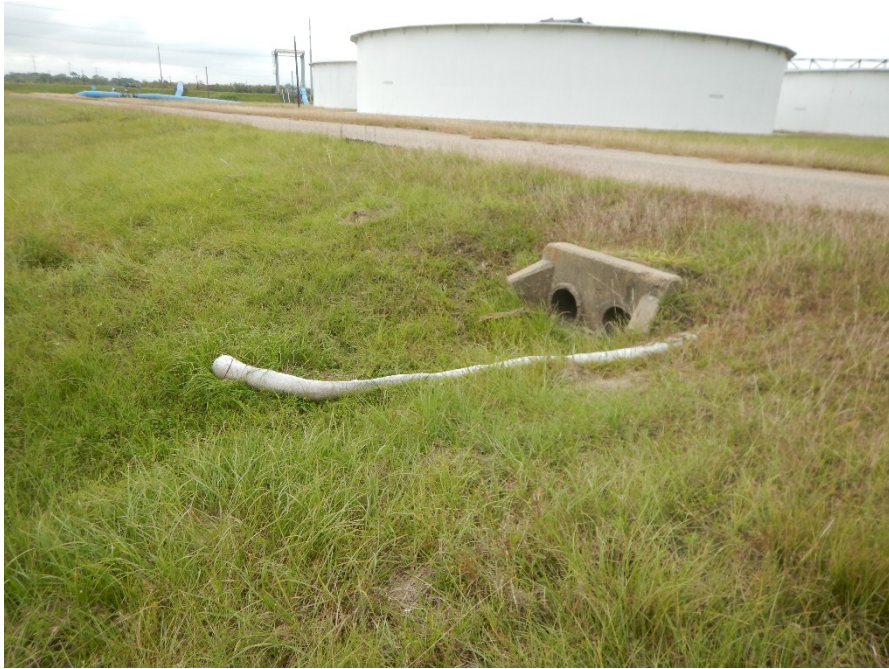
9. Outfall 003B discharge point
