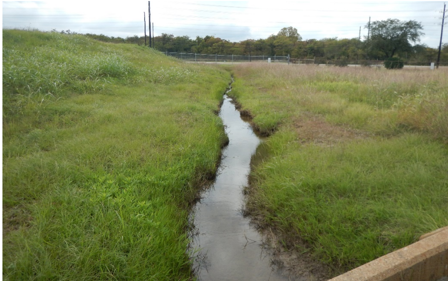
6. Outfall 003 looking downstream from outfall structure
