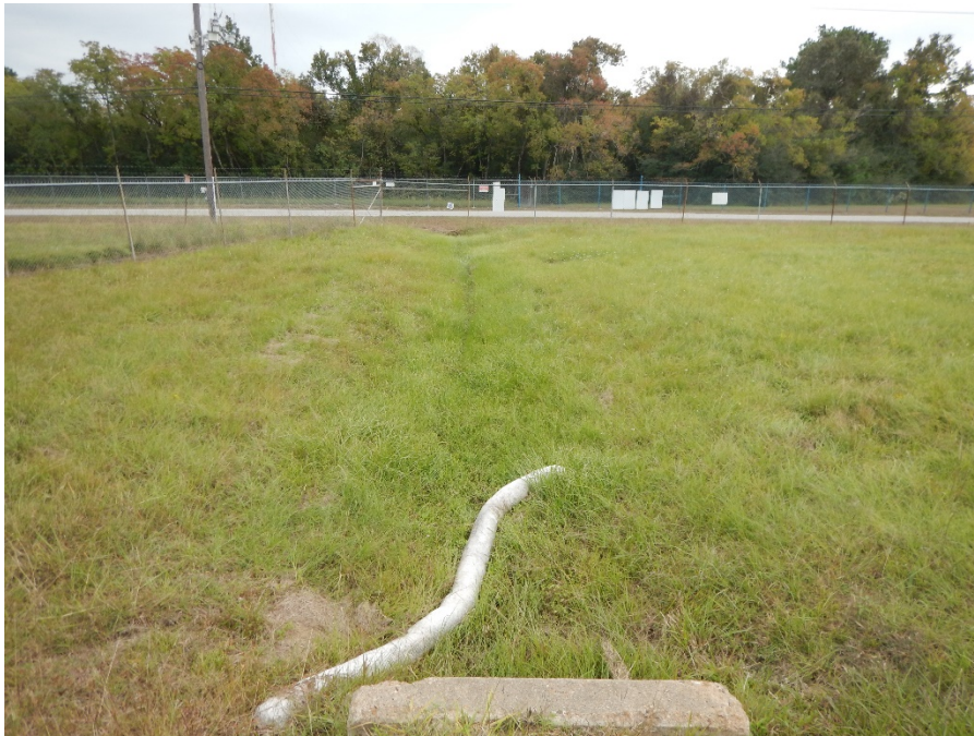
10. Outfall 003B looking downstream, outfall structure in bottom center
