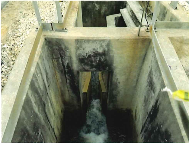
Photo 1. Outfall 001 at Parshall flume. Discharge exits to underground pipe.
