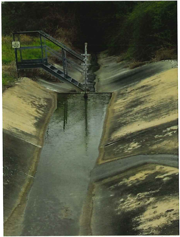
Photo 10. Outfall 006 at stairs, downstream in background.
