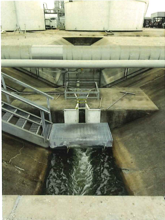
Photo 5. Outfall 004 at Parshall flume.
