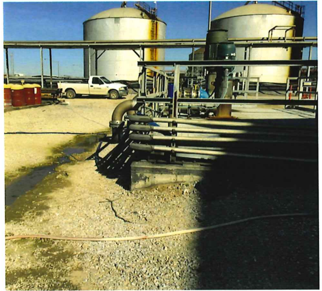
Photo 14. Outfall 009 (proposed), looking downstream at in-plant ditch.
