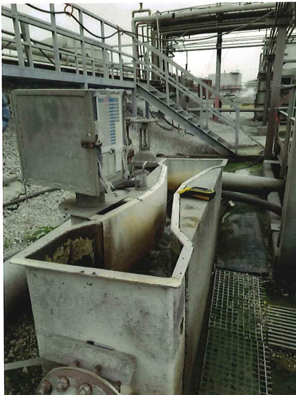
Photo 11. Outfall 007 at Parshall flume. Discharge exits to underground pipe.
