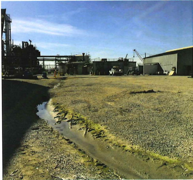
Photo 13. Outfall 009 (proposed), looking upstream at in-plant ditch.
