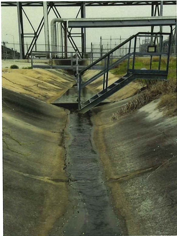
Photo 9. Outfall 006 at stairs, discharge in foreground.
