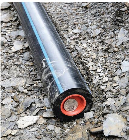
The quality of the 40 bar HDPE pipes is so convincing that they are laid directly into the trench without any additional precautions
