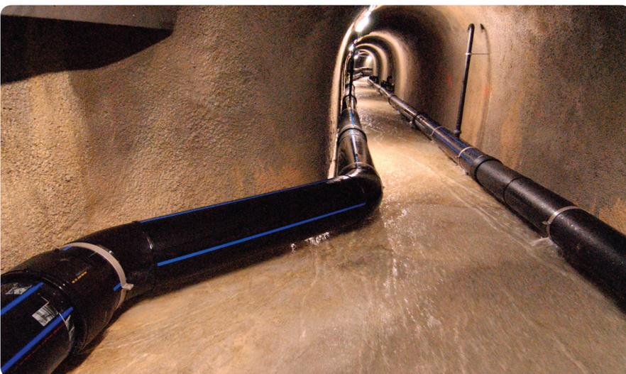
Shown here are the pipelines laid in the cavern area of the tunnel (N.B.: Depending on the weather conditions, there may at times be more water than the system can cope with. Surplus water, as in this photograph, then flows down through the tunnel and out into a stream)
