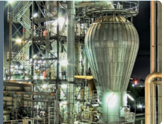
Spherilene process plant – LyondellBasell, Wesseling, Germany
